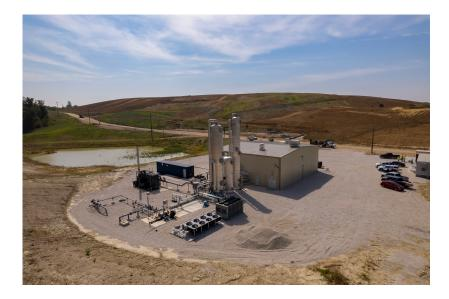
The plant processes about 1,500 standard cubic feet per minute of raw LFG and produces about 350,000 MMbtu per year of RNG. This is equivalent to producing 3,070,175 gallons of gasoline. The RNG can be used in a variety of energy and environmentally beneficial ways including:
